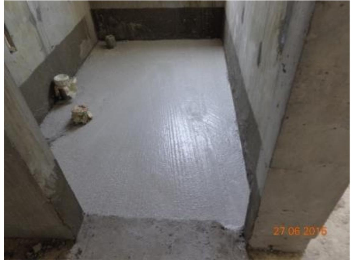
**TOWER F : Roof Completed and Internal Water Proofing Works in Progress**
